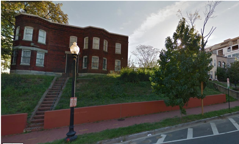
Figure 4. Petitioner's Property, from 2nd Street, NE
